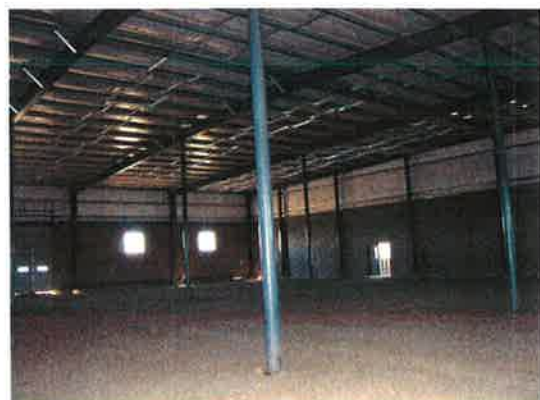
Photo B – Interior of Warehouse area (note no slab is installed).
