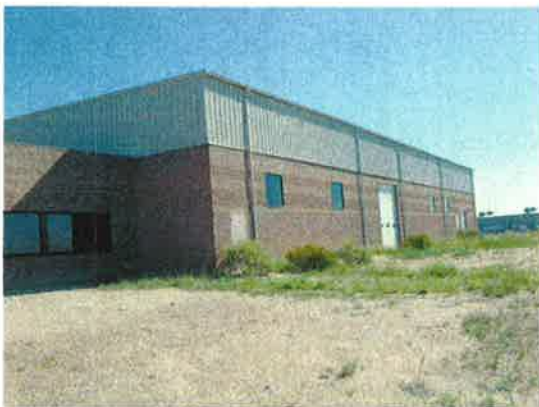
Photo A – Exterior of building looking northeast
